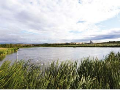
Dawson Creek Reclaimed Water Project
