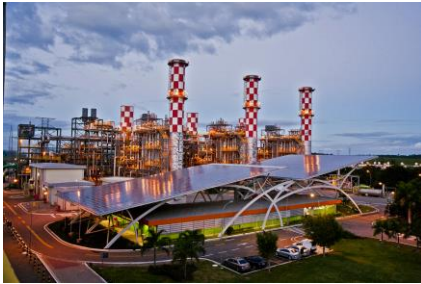
EDF Norte Fluminense CCGT (Photographer: João Salamonde)
