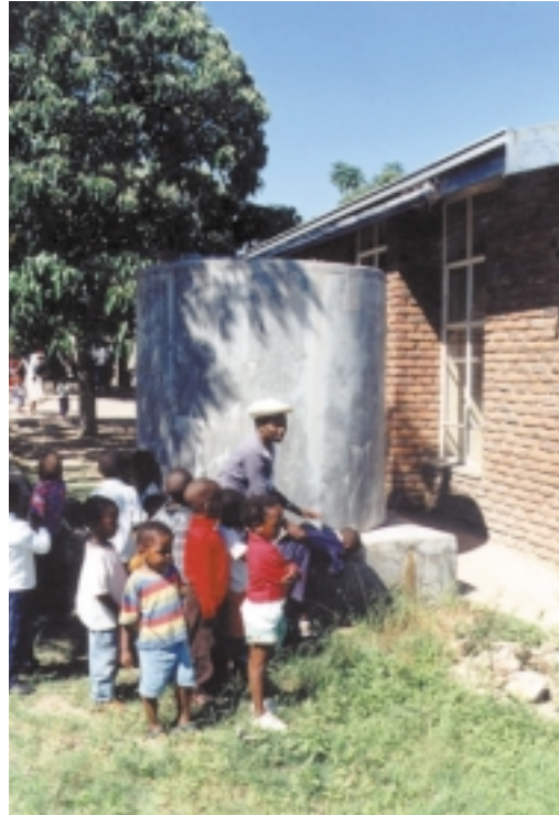
Water tank which captures rain water from roof tops
