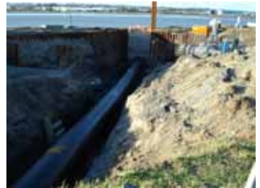
The 1,000-millimeter polyethylene pipe in position under the Whanganui River
