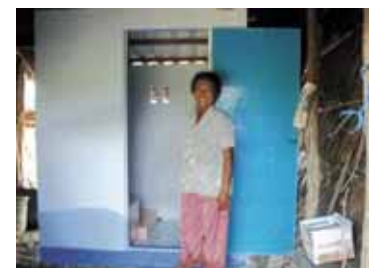
Examples of toilet buildings constructed by householders and community members
